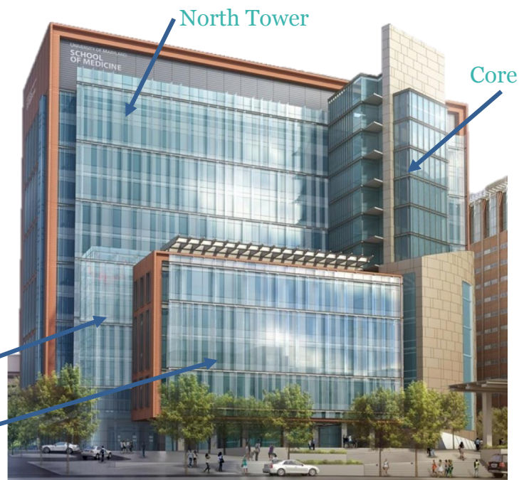
Figure 1: South view of HSFIII
